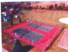
Summit Hill School Park Tennis Court Renovation
