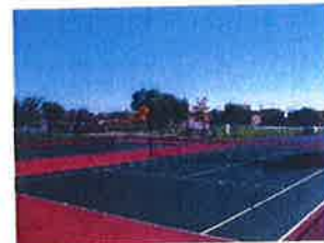
Community Park Tennis Court Renovation
