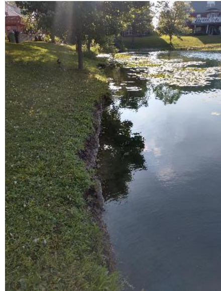
View of the erosion on the northern side of White Oak Park's northwestern basin.
